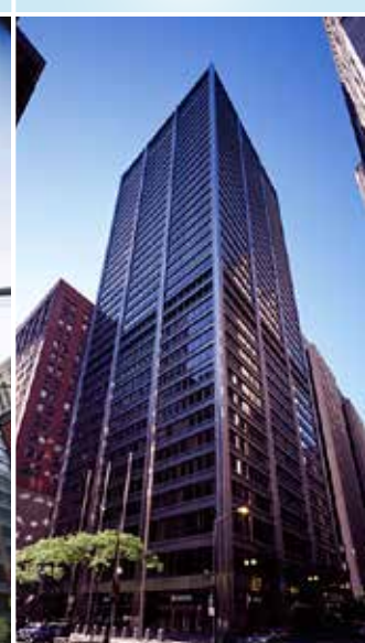
The Harris Bank Building - West
